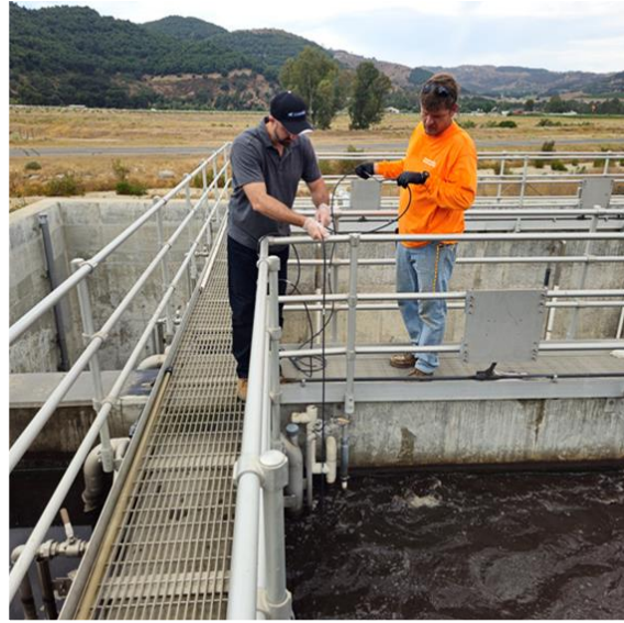
Establishing WWTP Probe Location
